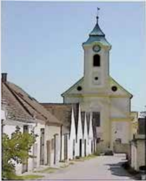
Burgenland, Oggau, Scheunensemble
